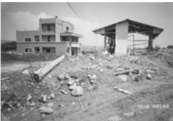
Photo 1: Flood damage at Mujiliao Village
