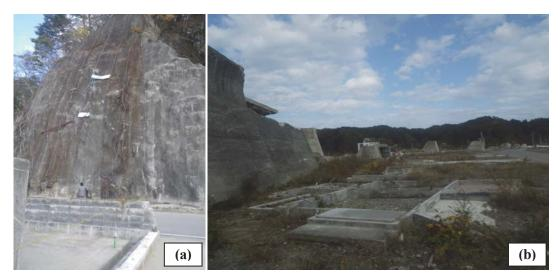
Figure 7. (a) Height records of historical tsunamis in 1896 (15 m) and 1933 (10 m) in Taro village (9/11/2011) and (b) destroyed seawalls (9/11/2011)
