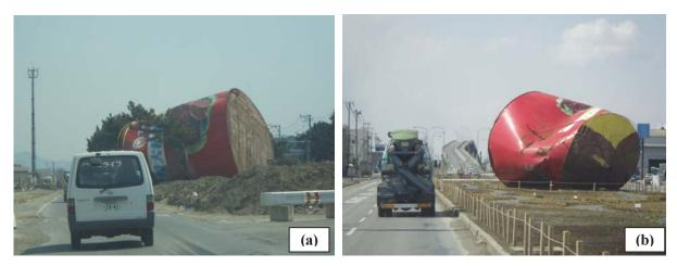
Figure 22. Large fish oil tank in Ishinomaki (a) after one month (15/4/2011) and (b) after one year (26/3/2012)
