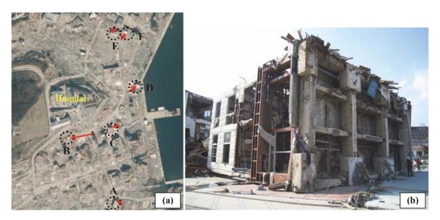
**Figure 20.** (a) Area map of Onagawa and location of its six overturned buildings A through F (6/4/2011), and (b) example of an overtopped building being saved for a memorial park (Building C) (29/3/2011)
