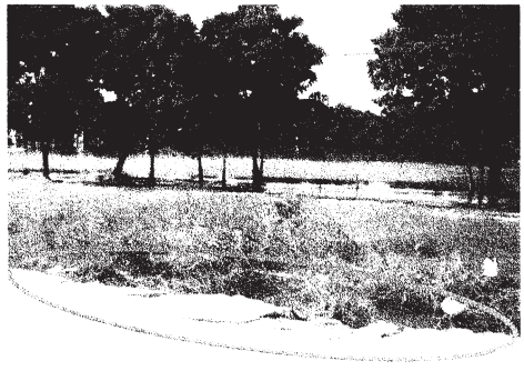
Photo 6 The road which was damage by the flood and the flood plain on the outskirts of Ang Thong city
