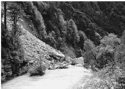
Photo 5 Channel blocked and ponded water at upper stream of Mo Chu (EL. 3,300m). Ponded water volume is approximately 1 \times 10^4 m^3 . Photo was taken on 14th September, 2009.
