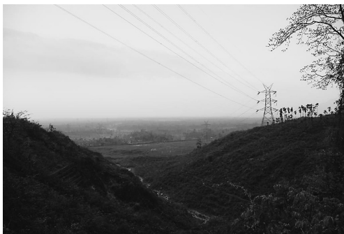
Photo 1 High voltage electric line ranges from Bhutanese mountain (near the side of photograph) to Indian plain. This is a typical scene of electricity export from Bhutan. Photo was taken in March, 2009.
