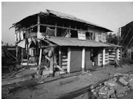
第8図 Damaged house near the Kuwakata coast
