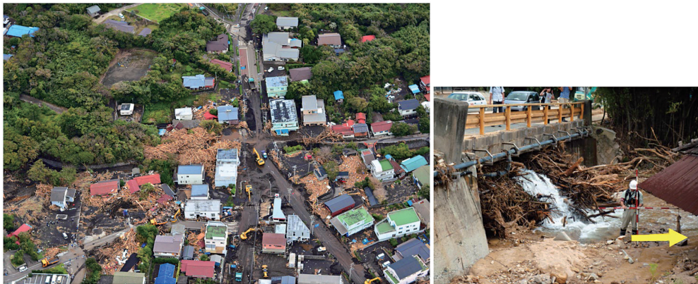
Photo 1. Bridges blocked with woody debris from debris flows: (left) Izu Oshima disaster (PASCO Co.) and (right) Houfu disaster (Furukawa et al. 2009).
